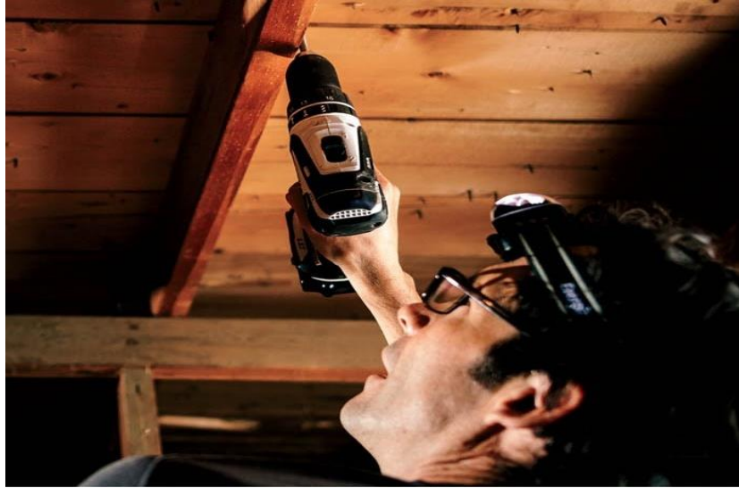
Gambar 6.3 Pengeboran lubang locator
