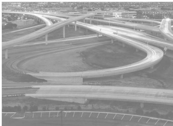
Gambar 6.6 Jembatan Girder Kotak Beton Melengkung—Persimpangan Rute 92/101, San Mateo, CA.
