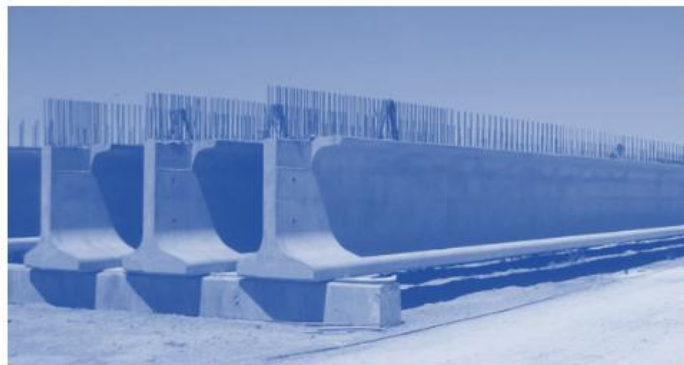
Gambar 1.2 Girder sayap lebar California.
