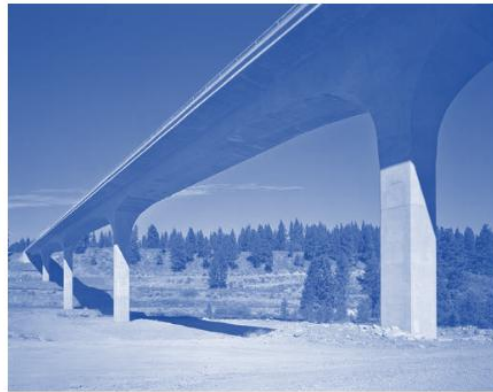
Gambar 2.7 Jembatan Sungai Truckee, California. (Courtesy of California Department of Transportation.)
