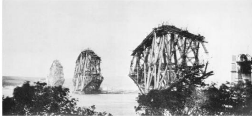
s. The massive cantilevers of the Forth bridge, shown under erection, were conceived in the shadow of the Tay bridge disaster.
