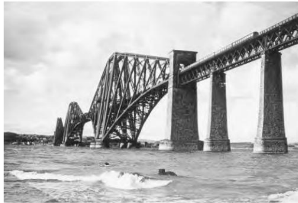
Gambar 3.2 Jembatan Firth Of Forth.
