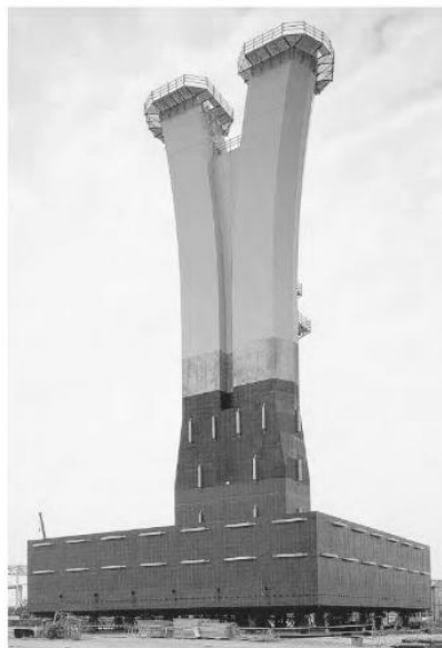
Gambar 4.48 Pilar Baja Berlapis Titanium.
