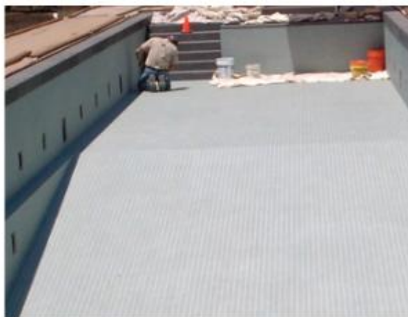
Gambar 3.3 Cangkang kolam renang baja berlapis ubin.
